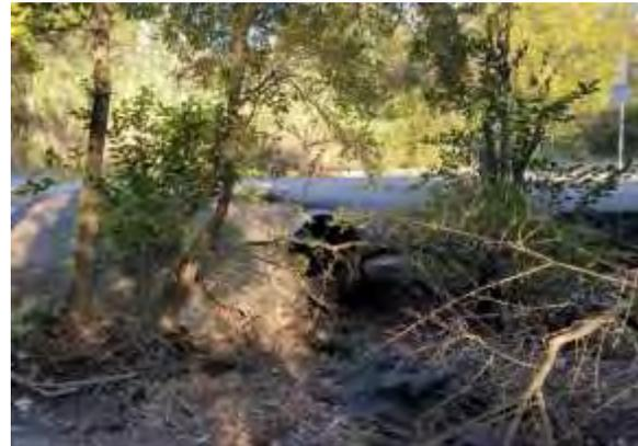
**Feature S-8** consists of a drainage culvert at the Eanes Creek tributary crossing of Camp Craft Road. It consists of a culvert approximately 4 feet wide that passes beneath the road surface, with grates on either side. The culvert is encased in concrete, and appears to extend into the bedrock of the creek channel. The culvert extends approximately 35 feet within the SITE.
