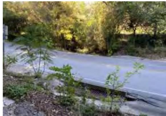
**Feature S-9** consists of a drainage culvert where Eanes Creek crosses beneath Eanes School Road. It consists of a rectangular concrete culvert with angular rock pieces enclosed in metal wire. The culvert is approximately 10 feet wide and 6 feet high and was installed beneath the bridge that crosses Eanes Creek on Eanes School Road. The culvert appears to extend into the bedrock of the creek channel and extends approximately 40 feet within the SITE.
