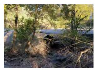
**Feature S-8** consists of a drainage culvert at the Eanes Creek tributary crossing of Camp Craft Road. It consists of a culvert approximately 4 feet wide that passes beneath the road surface, with grates on either side. The culvert is encased in concrete, and appears to extend into the bedrock of the creek channel. The culvert extends approximately 35 feet within the SITE.
