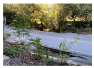
**Feature S-9** consists of a drainage culvert where Eanes Creek crosses beneath Eanes School Road. It consists of a rectangular concrete culvert with angular rock pieces enclosed in metal wire. The culvert is approximately 10 feet wide and 6 feet high and was installed beneath the bridge that crosses Eanes Creek on Eanes School Road. The culvert appears to extend into the bedrock of the creek channel and extends approximately 40 feet within the SITE.
