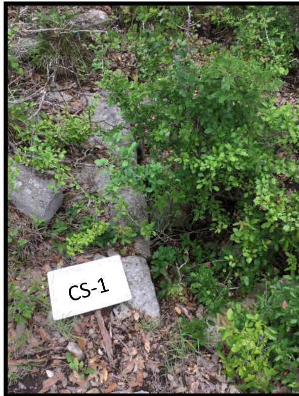
Feature CS-1: Sinkhole.
