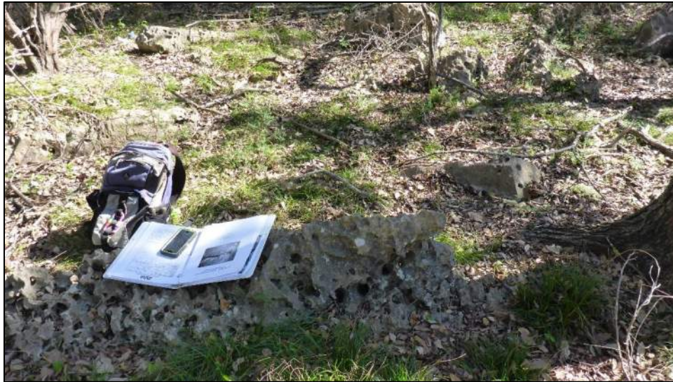
Figure 46. Overview of Feature R9 demonstrating typical honeycombed rock protruding from ground along the vuggy rock ridge.
