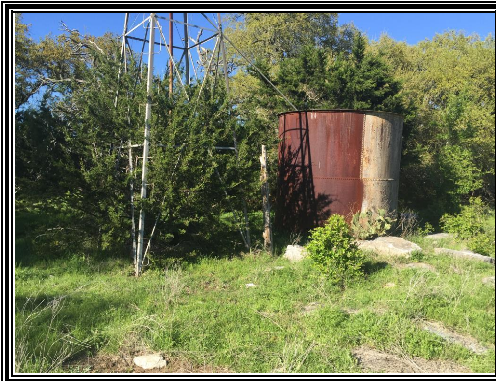
8. View of water well feature S-6, on the north-central portion of the site.
