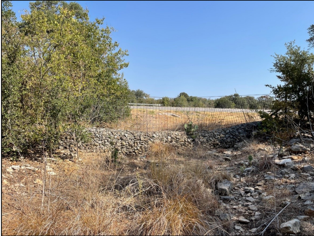
Photograph 3. Culvert overview near north end of project area.
