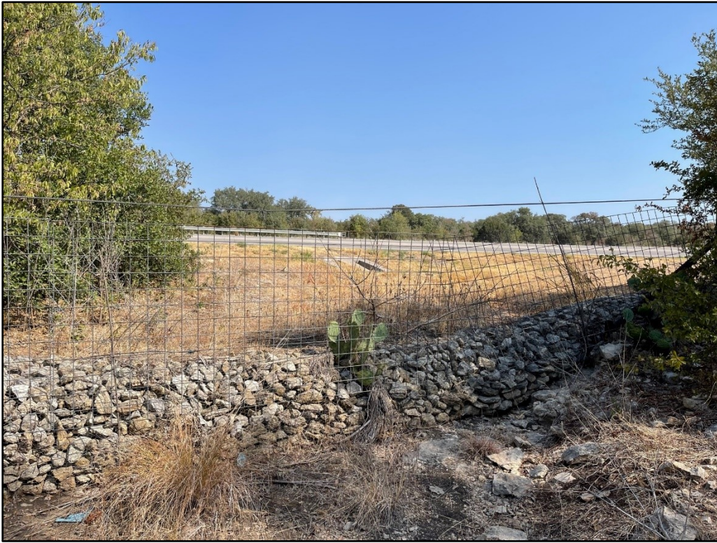
Photograph 1. Culvert located near north end of project area.
