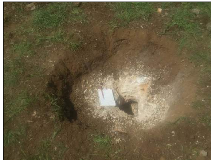
PHOTO 6 View of F-2A after hand excavation with open drainage portal
