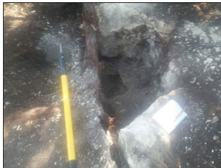
PHOTO 8 View of F-3 after hand excavation with no voids or open drainage portals
