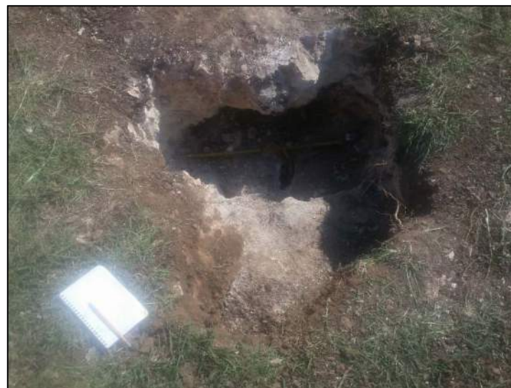
PHOTO 4 View of F-2 after hand excavation with open drainage portals
