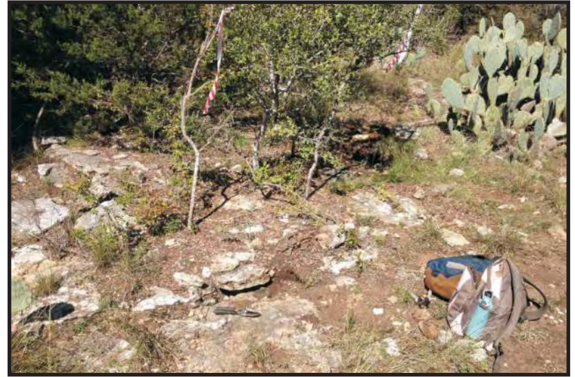
PHOTO 34 View of geologic feature F-21 (2 small solution cavities 8 ft apart), facing northwest
