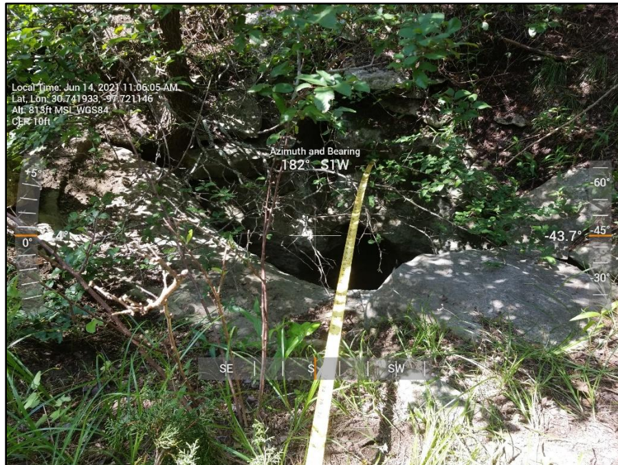
M-04 (View of depression)
