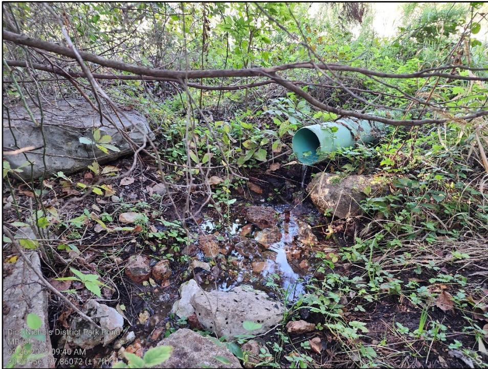
Figure 10. Water discharge pipe (MB-04) with pooling water.
