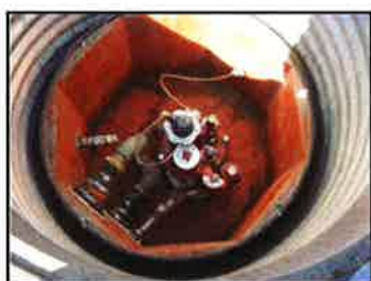
Dry, debris-free contained turbine sump
