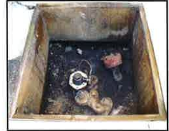
Uncontained turbine sump
