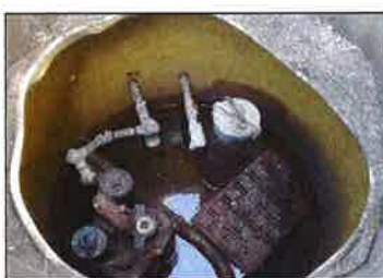
Contained sump with liquid and debris
