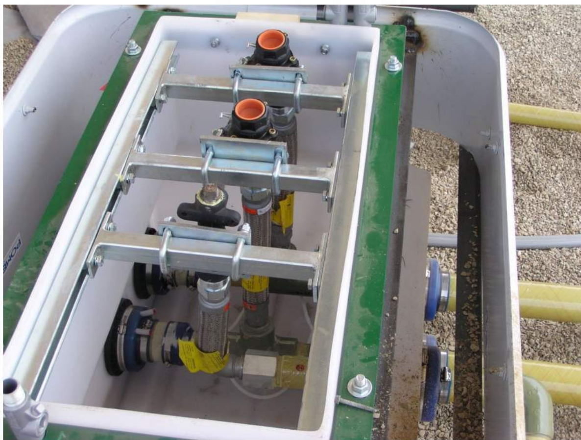
Figure 16. Photo of a Properly Anchored Shear Valve
