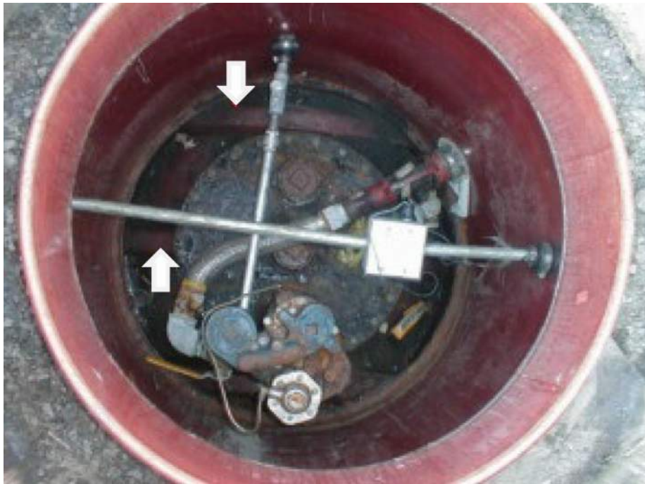
Figure 4. FRP Tank "Ribs" Seen Through Sump Opening
