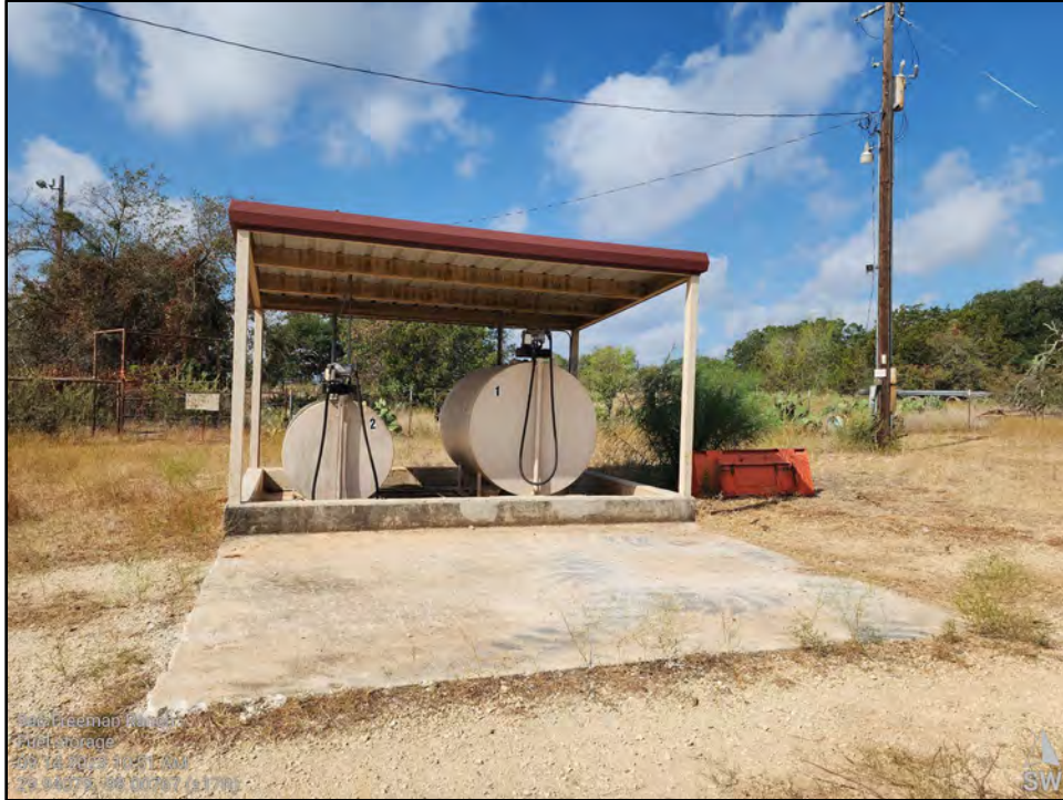
Figure 6. Fuel storage area with two ASTs and secondary containment located northeast of the Project Area.
