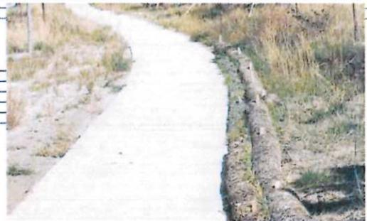
When installing in a channel bottom, AEC Premier Straw Wattle installation shall continue three feet above the anticipated high water mark.
