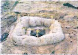
Curlex Sediment Logs use excelsior fibers to reduce hydraulic energy & filter sediment-laden runoff. Tired of straw and hay bale checks being blown out and the fibers washed downstream to clog the nearest outlet? Fed up with spending all of your time and effort installing silt fence only to see it get knocked down when it rains or a good wind comes along? How about when you have to go back and pick up the loose fibers and/or remove those worn out silt fences and take them to the landfill?
