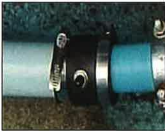
Test boot located in a sump
