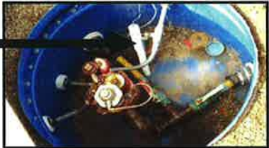
Sump sensor in contained turbine sump
