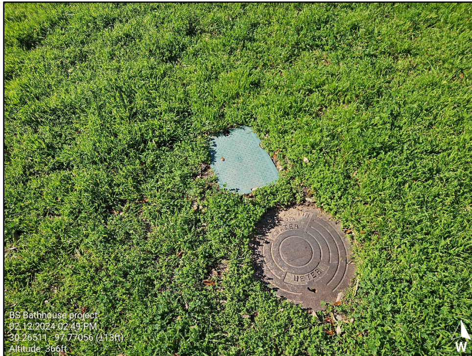
Figure 7. Example of water main infrastructure associated with MB-02.
