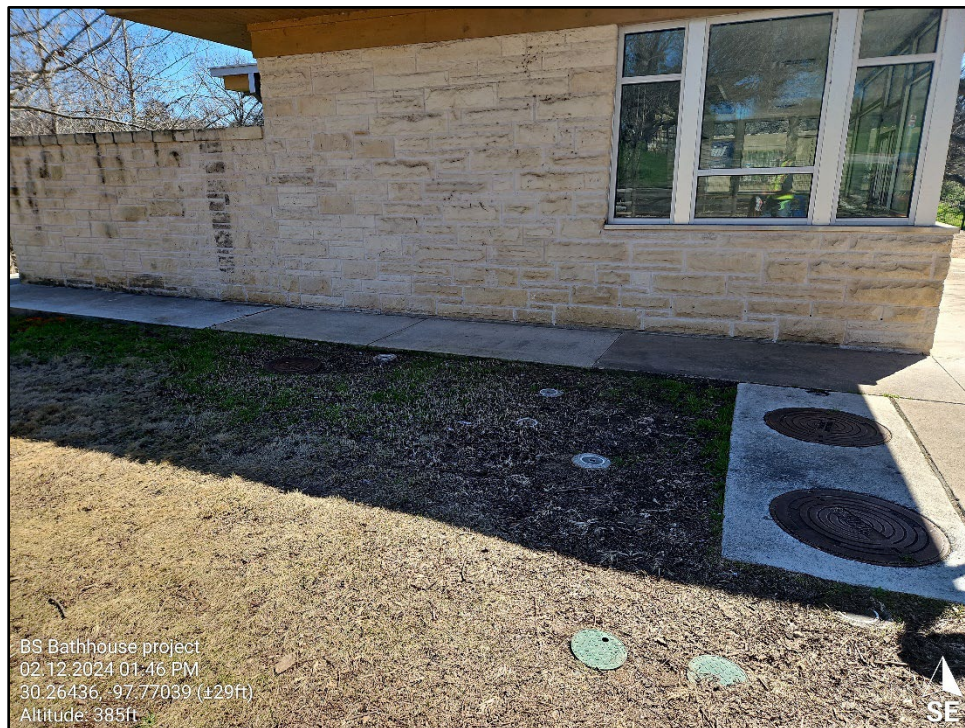
Figure 8. Example of wastewater infrastructure associated with MB-03.
