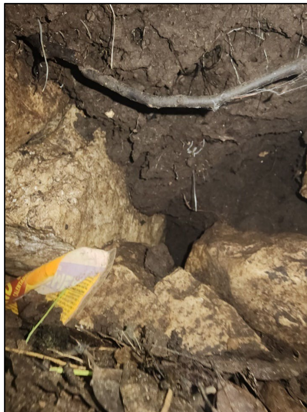
Figure 12. Interior of BS-01.
