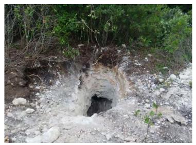
PHOTO 19 View of geologic feature F-16 (sinkhole/solution-enlarged fracture) after mechanical excavation, facing north
