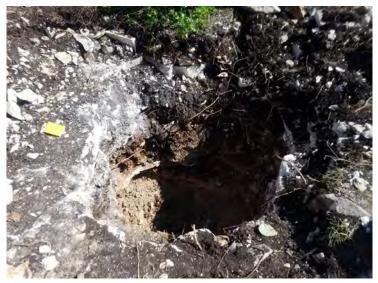
PHOTO 22 View of geologic feature F-19 (solution-enlarged fracture) after mechanical excavation, facing down
