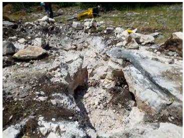
PHOTO 17 View of geologic feature F-14 (sinkhole) after mechanical excavation, facing north
