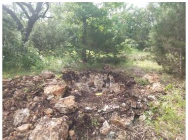
PHOTO 25 View of geologic feature F-22 (solution cavity) after mechanical excavation, facing south
