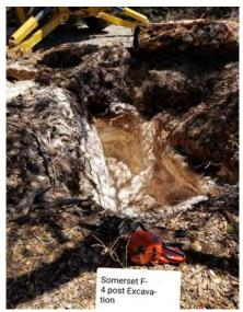
PHOTO 1 View of geologic feature F-4 (solution cavity) after mechanical excavation, facing down
