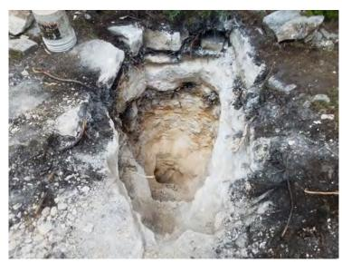
PHOTO 27 View of geologic feature F-24 (sinkhole/solution-enlarged fractures) after mechanical excavation, facing down
