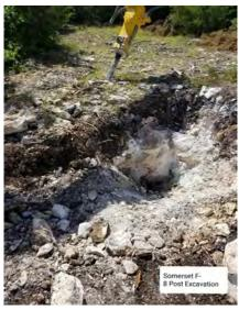
PHOTO 6 View of geologic feature F-8 (upland sinkhole) after mechanical excavation, facing north
