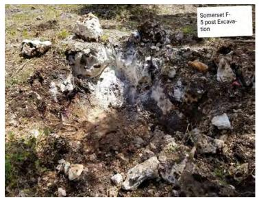
PHOTO 2 View of geologic feature F-5 (solution cavity) after mechanical excavation, facing down
