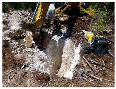
PHOTO 18 View of geologic feature F-15 (solution cavity) after mechanical excavation, facing north
