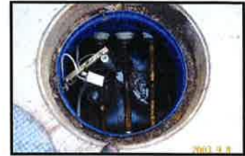
Transition/intermediate sump
