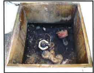
Uncontained turbine sump
