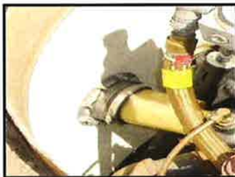
Sump penetration seals in good condition
