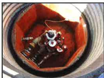
Dry, debris-free contained turbine sump
