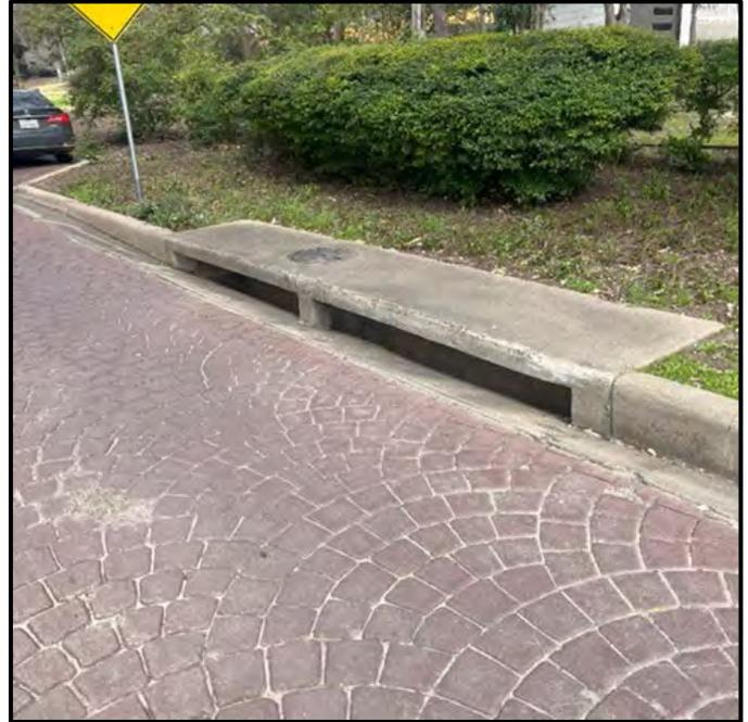
Photo 18. Stormwater inlet on east side of Las Lomas Dr. Looking east.
