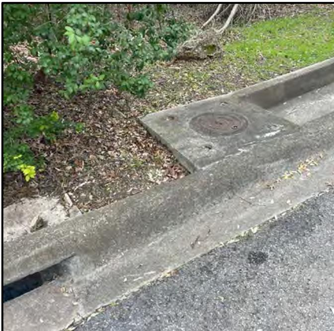
Photo 39. Concrete channel on west side of Cedar Park Drive that runs into stormwater inlet. Looking west.
