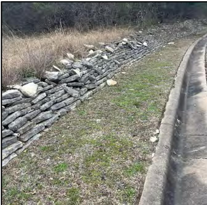
Photo 27. Limestone rock retaining wall along southern project area of Bent Tree Ct.
