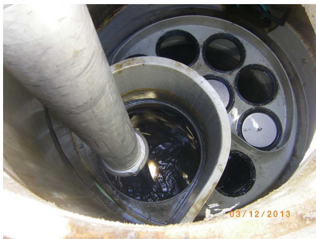
A maintenance worker stationed on the surface uses a vacuum hose to evacuate water, sediment, and floatables from the Jellyfish Filter by inserting the vacuum wand through the maintenance access wall opening.
