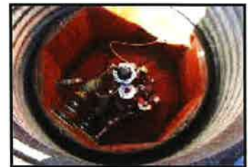
Contained turbine sump
