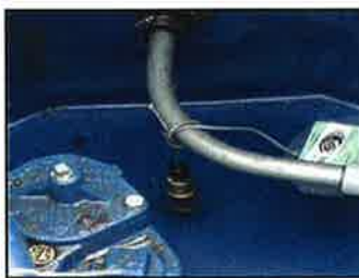
Liquid sump sensor
