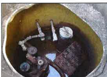
Contained sump with liquid and debris
