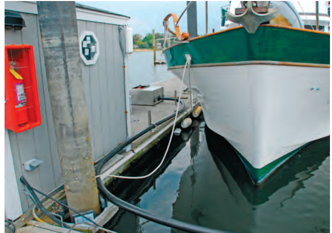
Connection to the dispenser sump
