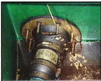
Sump penetration seals in poor condition
