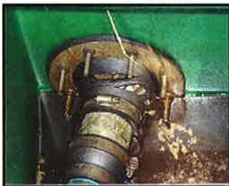
Sump penetration seals in poor condition
