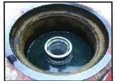
Spill bucket that contains liquid
