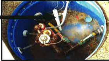
Sump sensor in contained turbine sump
