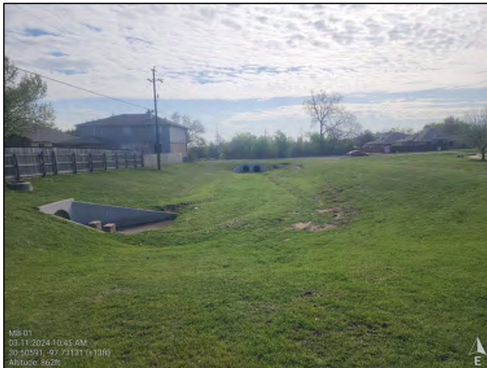
Figure 4. Overview of MB-01, a stormwater ponding basin.
