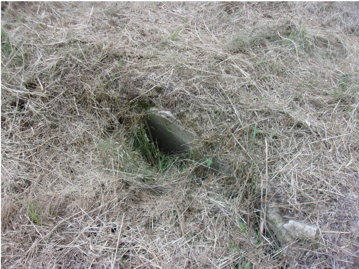
6. Internal wall of hand dug well
