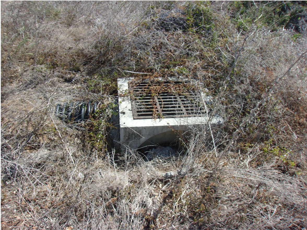
5. Storm drain inlet on east central portion of site
