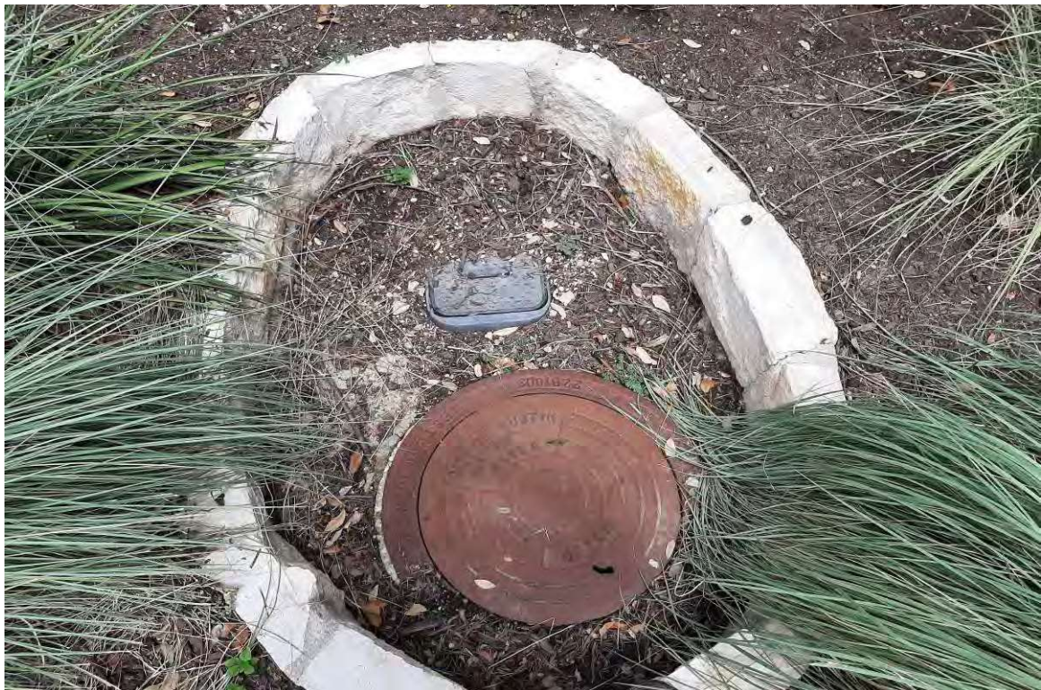
Photo 10. MB-006, City of Austin meter and shut off
