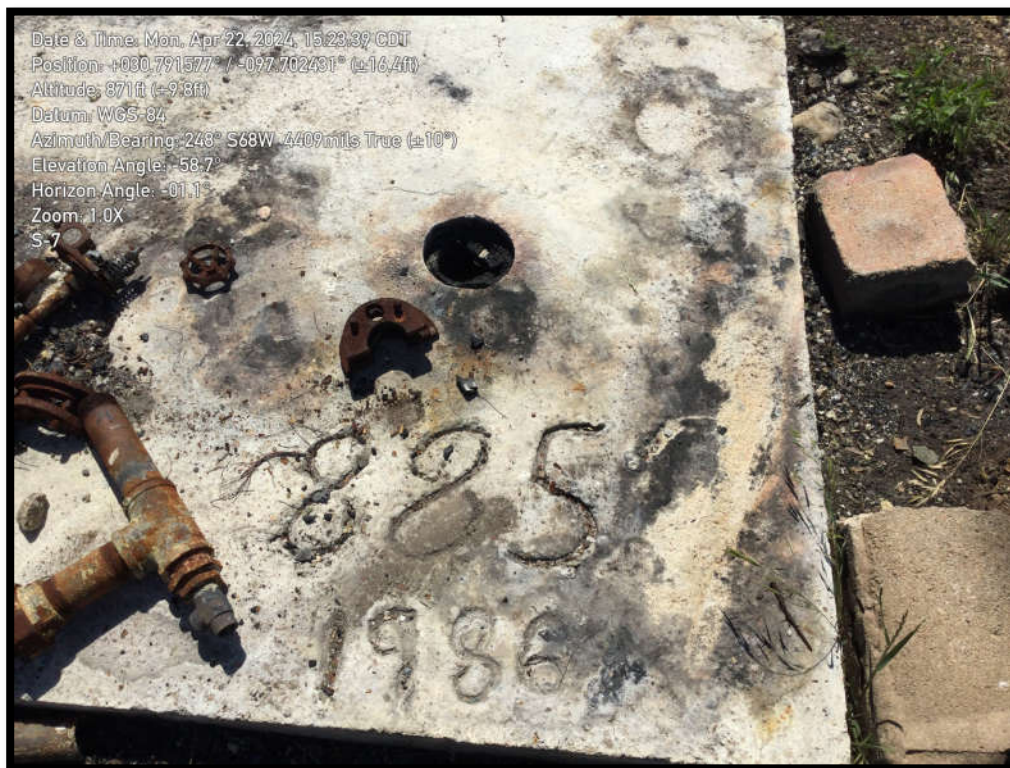
S-7: Open well with possible indication of total depth and year completed.
