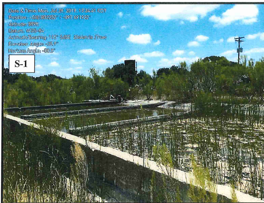
S-1 Tanks holding water within the southeast corner of the main pit, view to the southeast.
