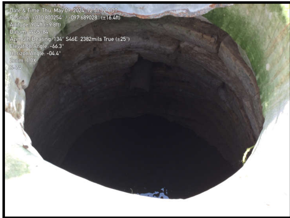
S-74: View down the cistern.
