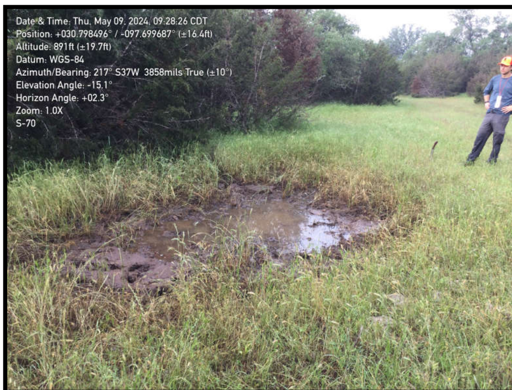
S-70: Non-karst closed depression located on the western part of the Site.
