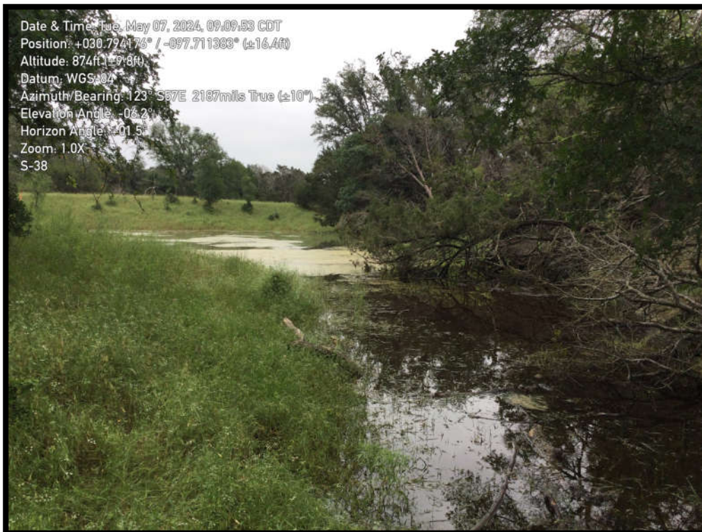
S-38: Non-karst closed depression created by dam on the western part of the Site.
