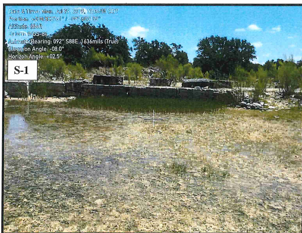
S-1 Standing water in northern area of main pit, view to the east.
