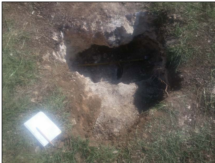
PHOTO 4 View of F-2 after hand excavation with open drainage portals
