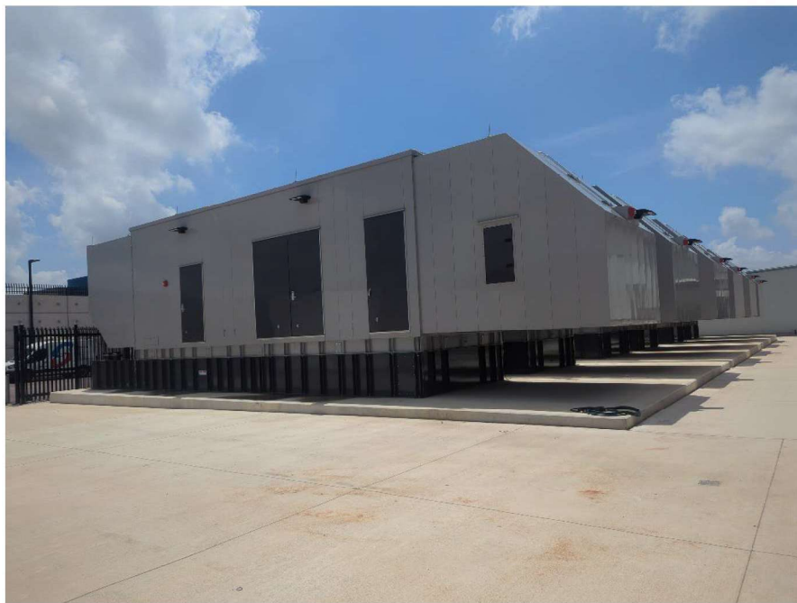
Representative photo of the concrete pads, emergency generators, and above ground storage tank areas.
