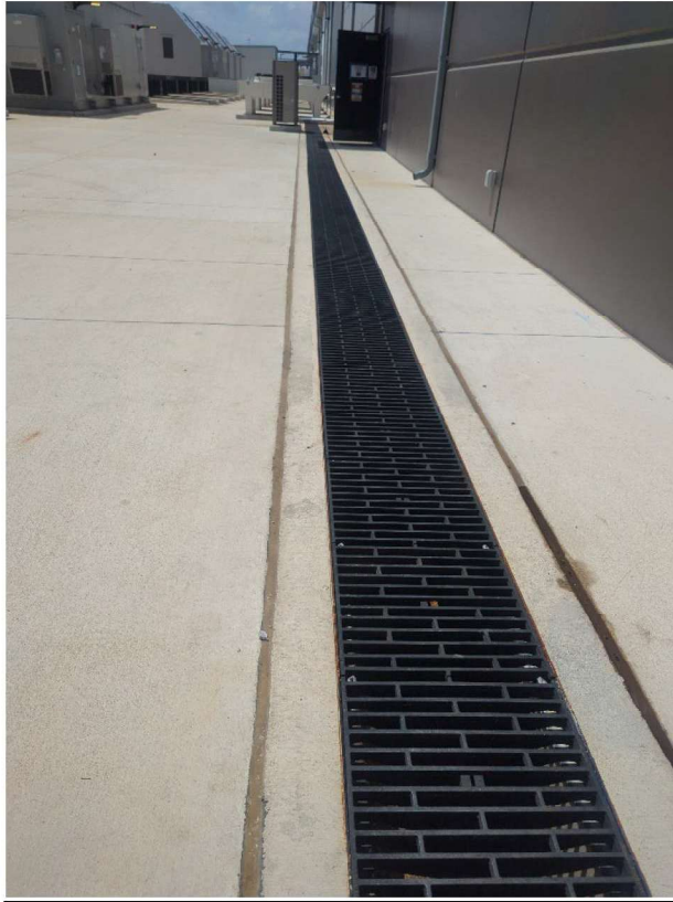
Representative photos of the concrete and storm drain system situated between the Switch Data Center building and the emergency generators and above ground storage tank areas.
