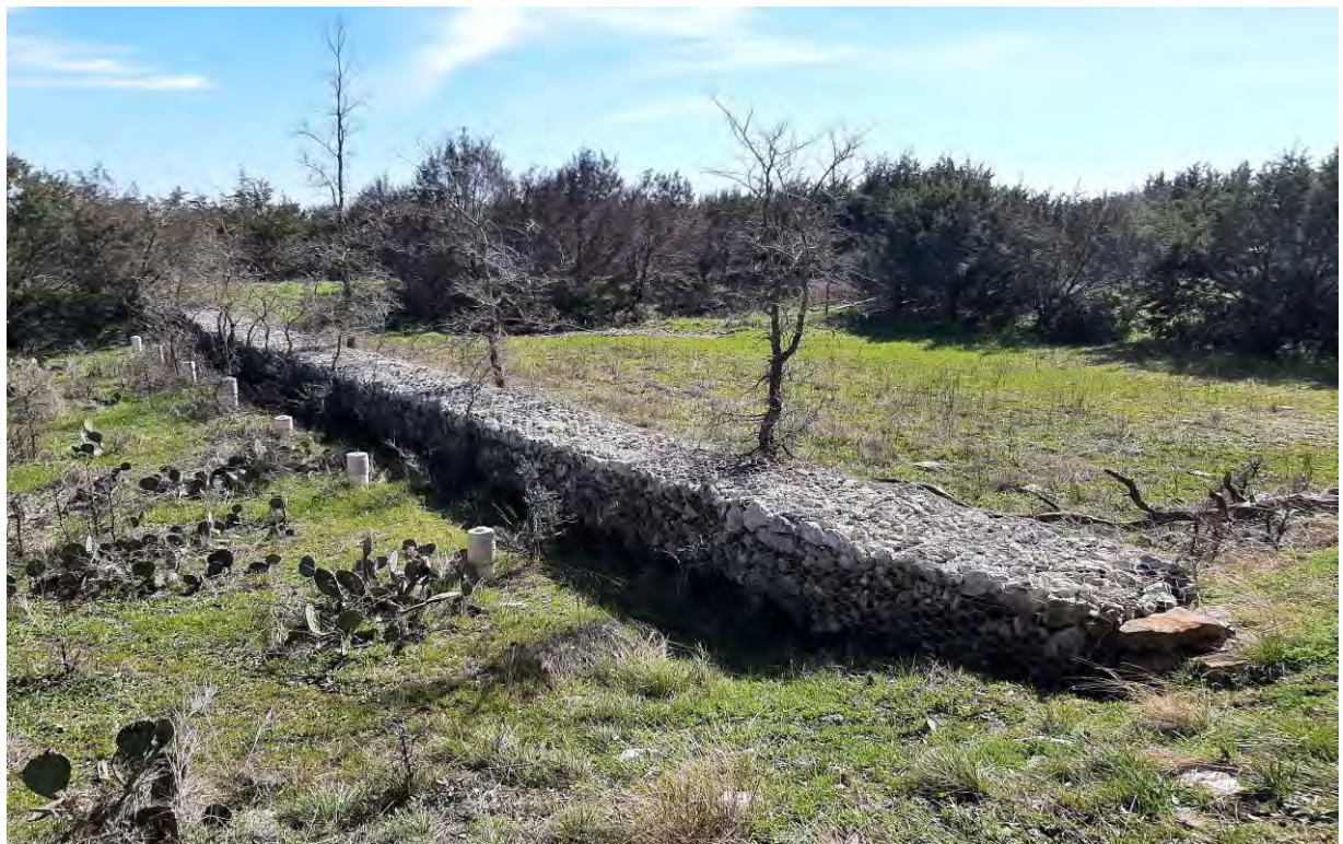
Photo 4. D-1, First stage detention, facing east.
