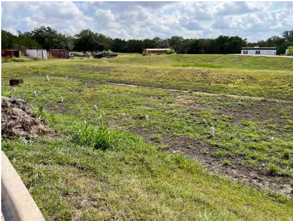
Photo 4 – View of a stormwater quality pond located east of the Fire Training Tower. View to the northeast.
