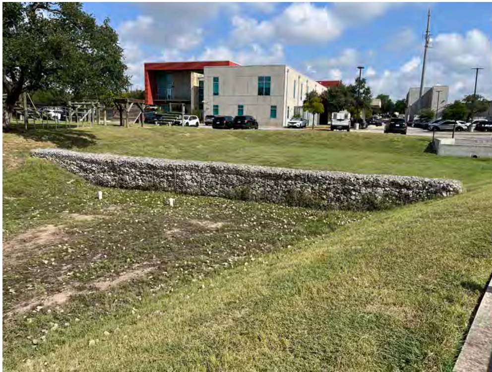
Photo 3 – View of a stormwater quality pond located south of the Public Safety Operations Building. View to the north.
