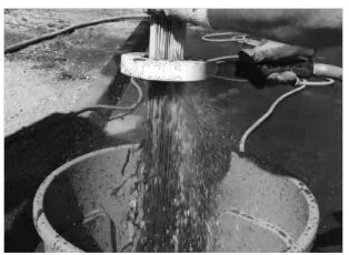
Pressure wash cartridge deck and receptacles to remove all sediment and debris. Sediment should be rinsed into the sump area. Take care not to flush rinse water into the outlet pipe. 4. Remove water from the sump area. Vacuum or pump
