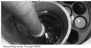
vaults complete sediment removal may be facilitated by removing a cartridge lid from an empty receptacle and inserting a jetting wand (not a vacuum wand) through the receptacle. Use the sprayer to rinse loosened sediment toward the vacuum
