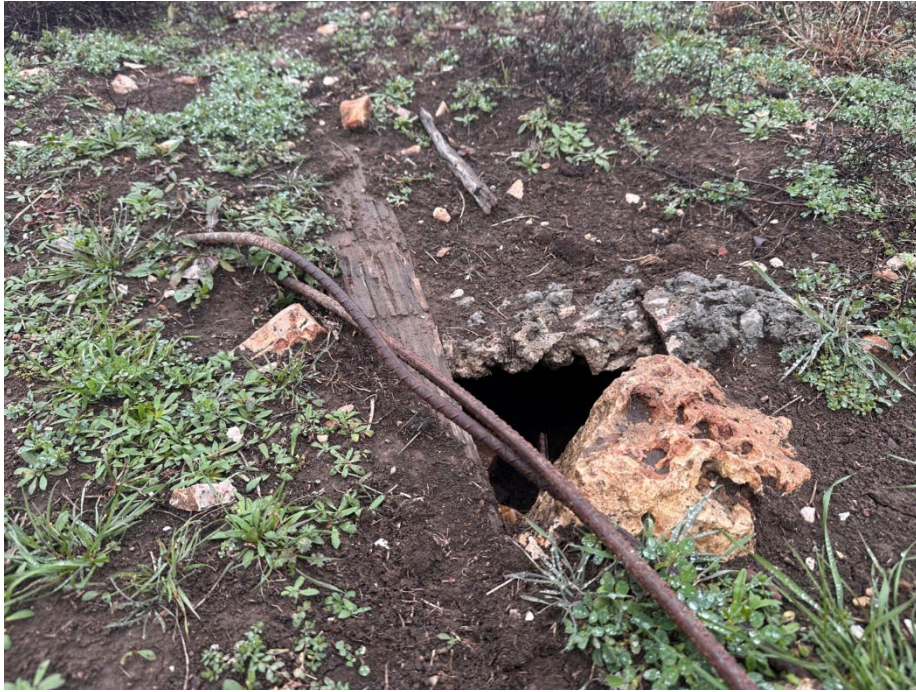
Photo 5 View of the area of disturbance characterized as a former excavation backfilled with soil, rock, and debris consisting of timber, iron rebar, and concrete.
