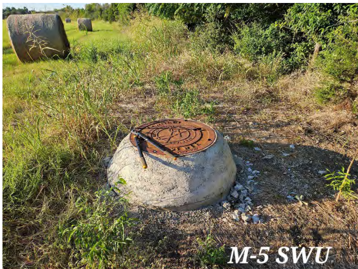
PHOTO 7 Man-made feature M-5 (sanitary sewer manhole)
