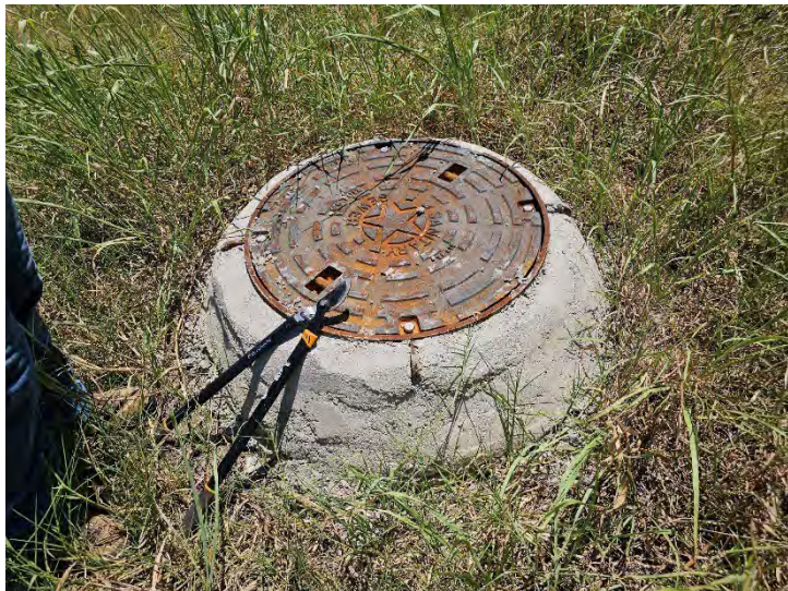
PHOTO 5 Man-made feature M-3 (sanitary sewer manhole)
