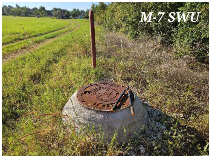
PHOTO 9 Man-made feature M-7 (sanitary sewer manhole)
