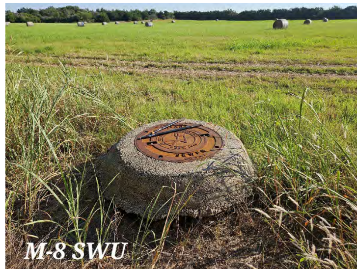
PHOTO 10 Man-made feature M-8 (sanitary sewer manhole)
