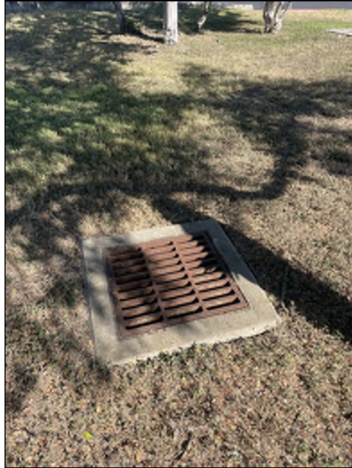
3 - Stormwater inlet observed in grassy area adjacent to south parking lot.
