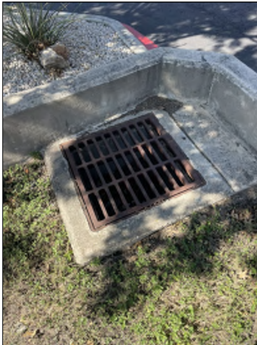
18 - Stormwater inlet on south portion of the property.
