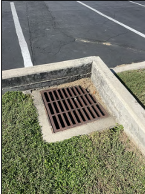
17 - Stormwater drainage inlet observed on the south portion of the property.
