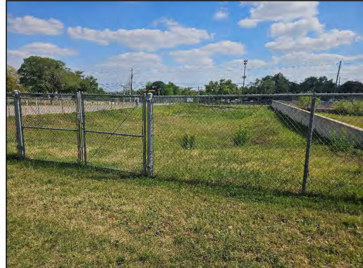
PHOTO 10 View of man-made feature M-3, facing southeast
