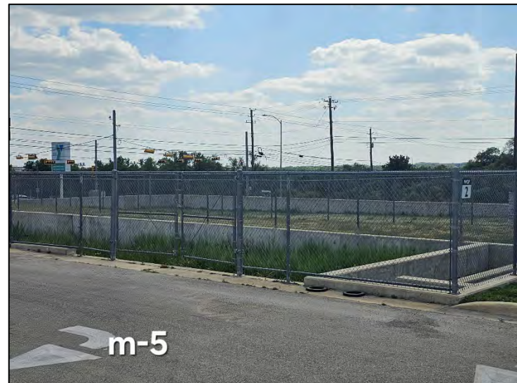
PHOTO 12 View of man-made feature M-5, facing southwest
