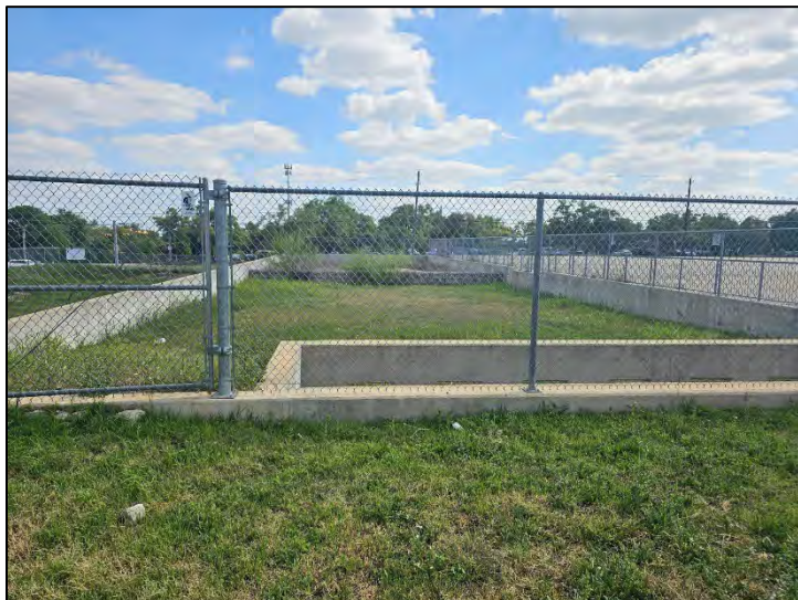
PHOTO 11 View of man-made feature M-4, facing southeast
