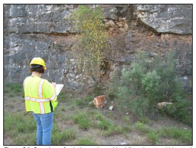
Figure 94. Overview of solution-enlarged bedding plane and bisected solution cavity added to the feature 1604-F070 description.
