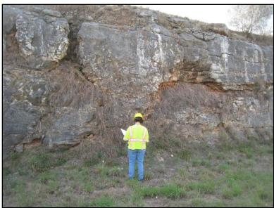
Figure 228. Overview of feature 1604-T12. The sinkhole is on the left and the solution-enlarged bedding plane on the right.
