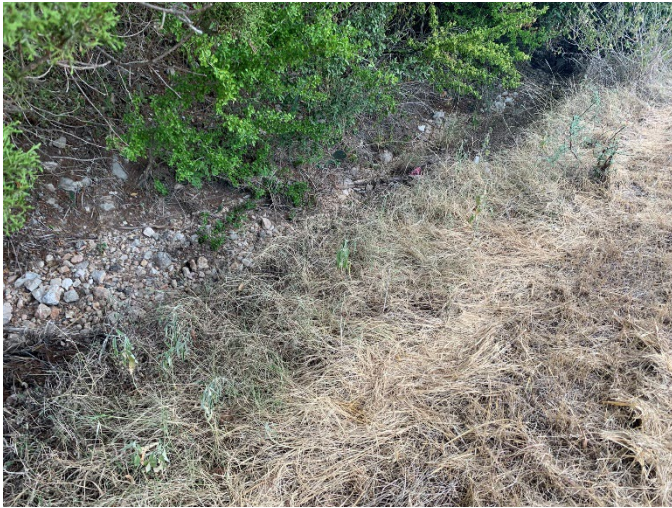
Western Site Drainage
