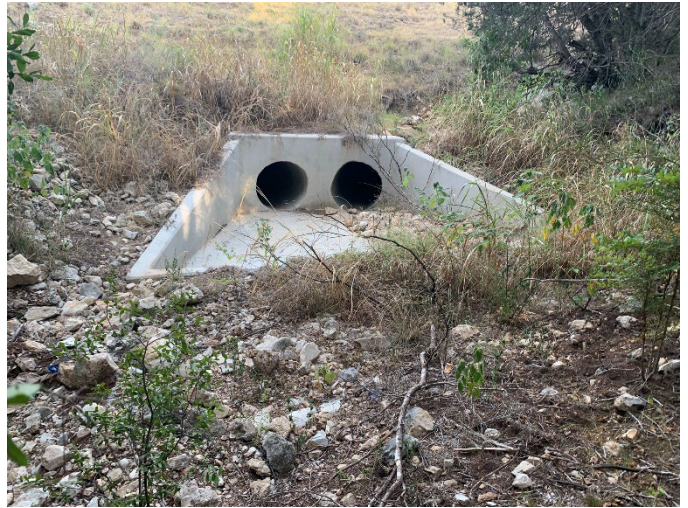
Culvert Draining Site Where Western and Eastern Site Drainages Converge
