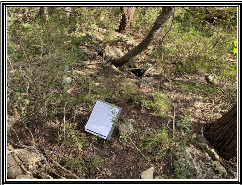
6. View of solution cavity feature S-3, located at 29-42-33.8 98-9-56.6, in the uplands on the North Tract, in the southwest portion.
