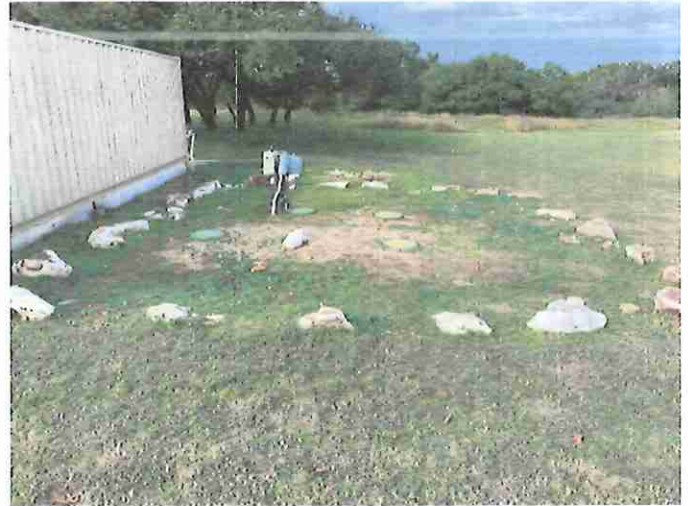
Area of S-102 Manmade Feature in Bedrock (Septic System) from 2013 Frost Geologic Assessment (Unable to Locate)
