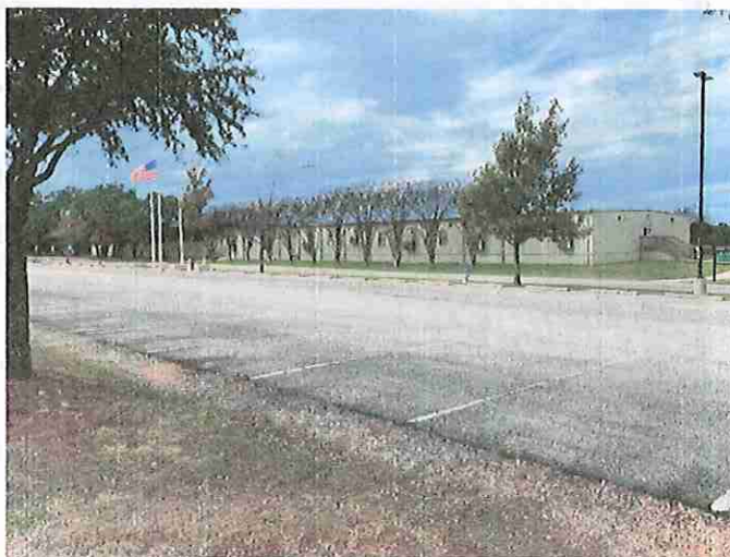
Front Parking Lot Area and Classroom Buildings
