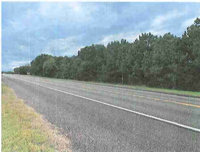
Site Southern Corner
