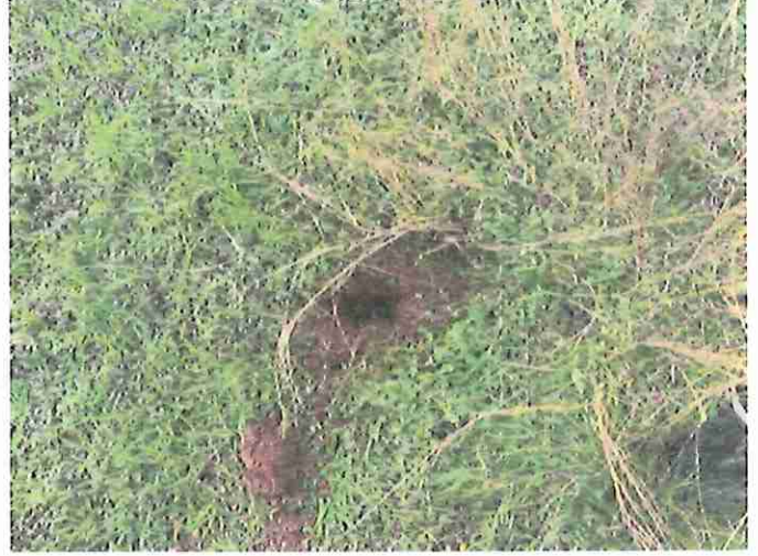
CD-1 – Non-Karst Closed Depression within Manmade Berm
