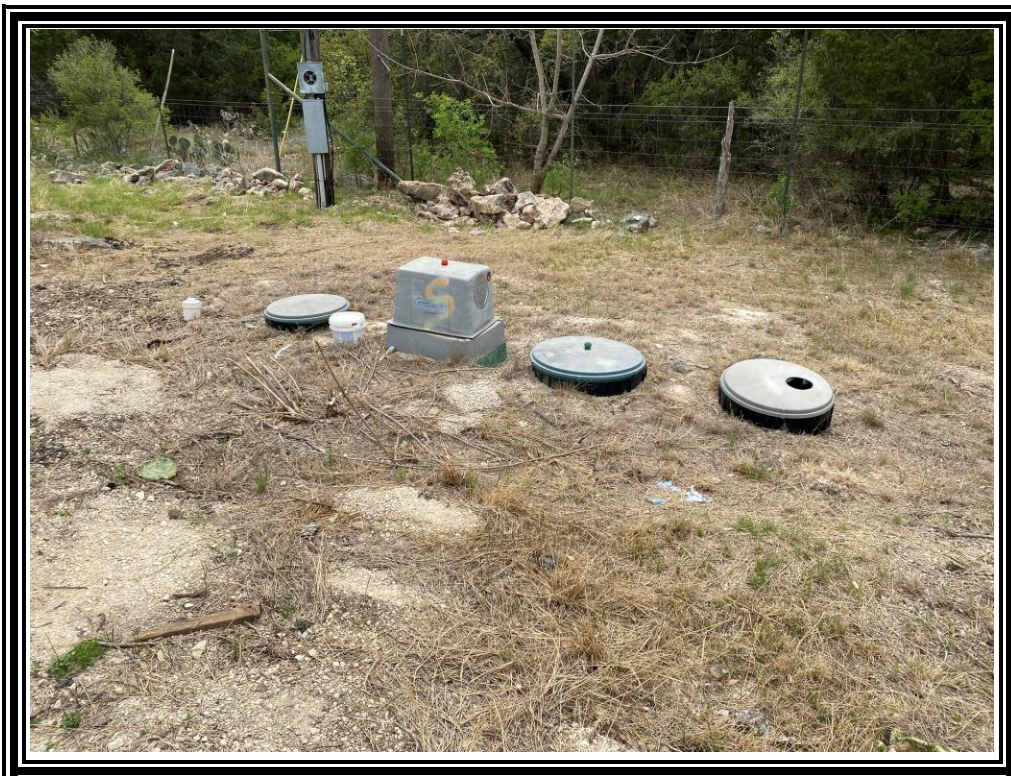
6. View of septic tank Feature S-2 located near the west corner.
