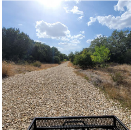
View to the west of the project site near PRF #S-513.
