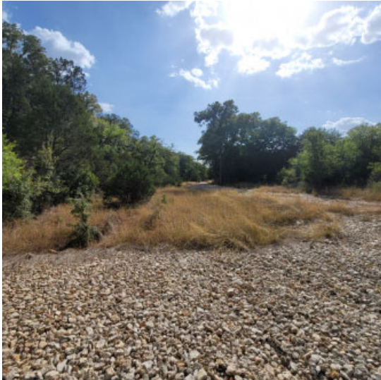
View to the southwest of the project site near PRF #S-522.
