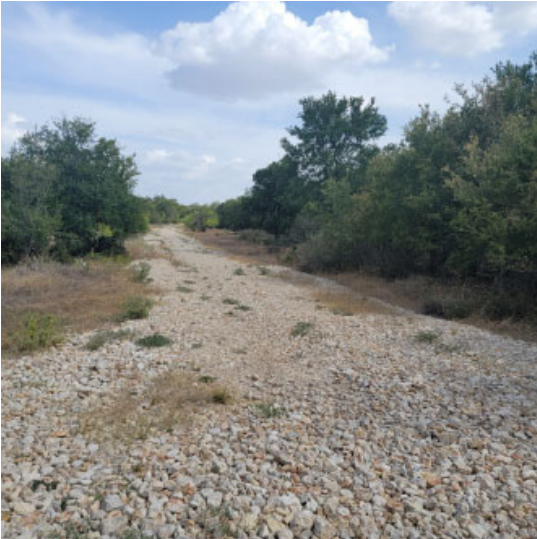
View to the southeast of the project site near PRF #S-506.
