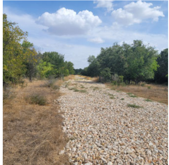
View to the southeast of the project site near PRF #S-505.
