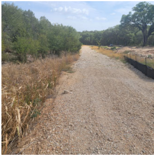
View to the south of the project site near PRF #S-501.
