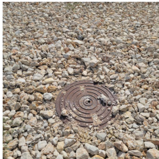
View of Potential Recharge Feature # S-506.
