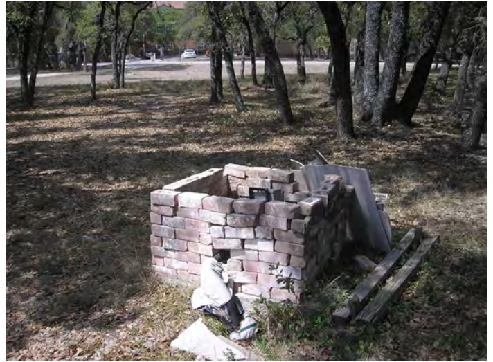
Photo #14 – View of a brick enclosure containing PRF #S-10.
