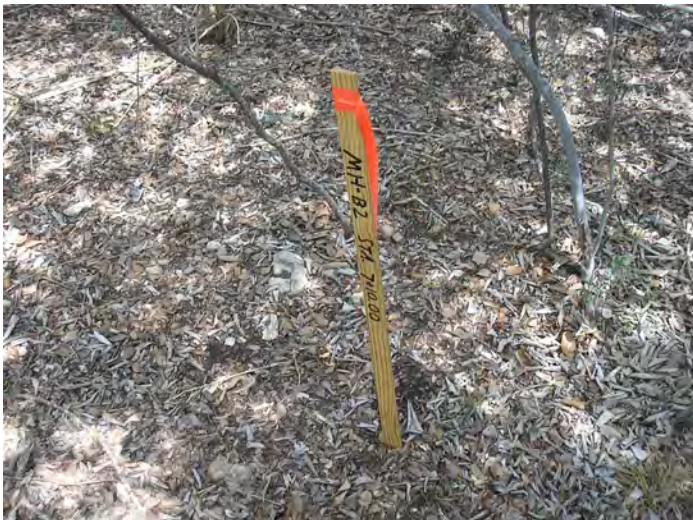
Photo #23 – View of survey stake marking the location of a proposed sanitary sewer manhole.
