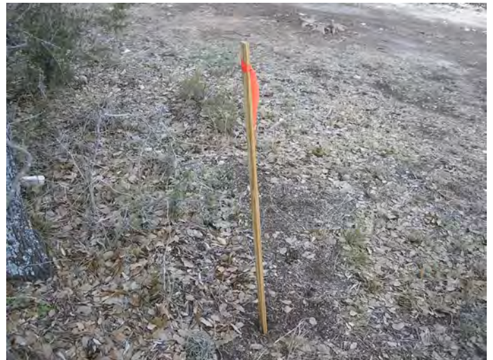
Photo #24 – View of an additional survey stake marking the location of a proposed sanitary sewer manhole.
