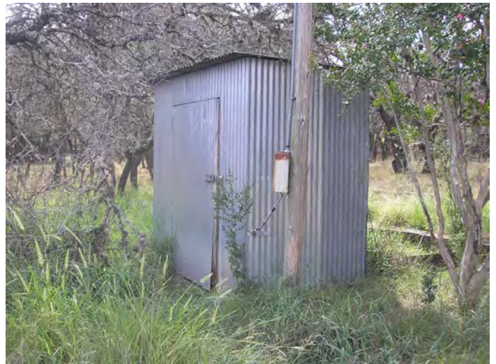
Photo #8 – View of the shed containing PRF # S-4.
