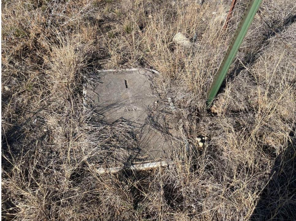
Photo #12: View of AT&T communication manway box at the location of feature S-5.
