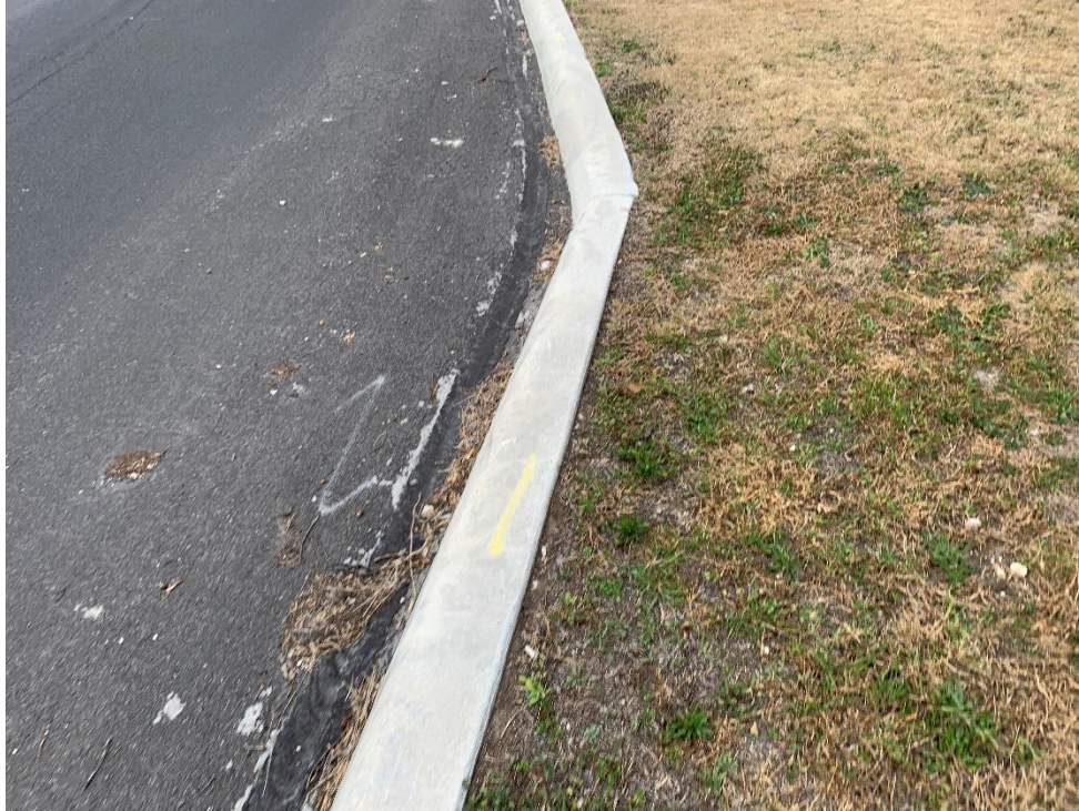
Photo #12: View of marked gas line at the location of feature S-8. Photo taken January 6, 2023.
