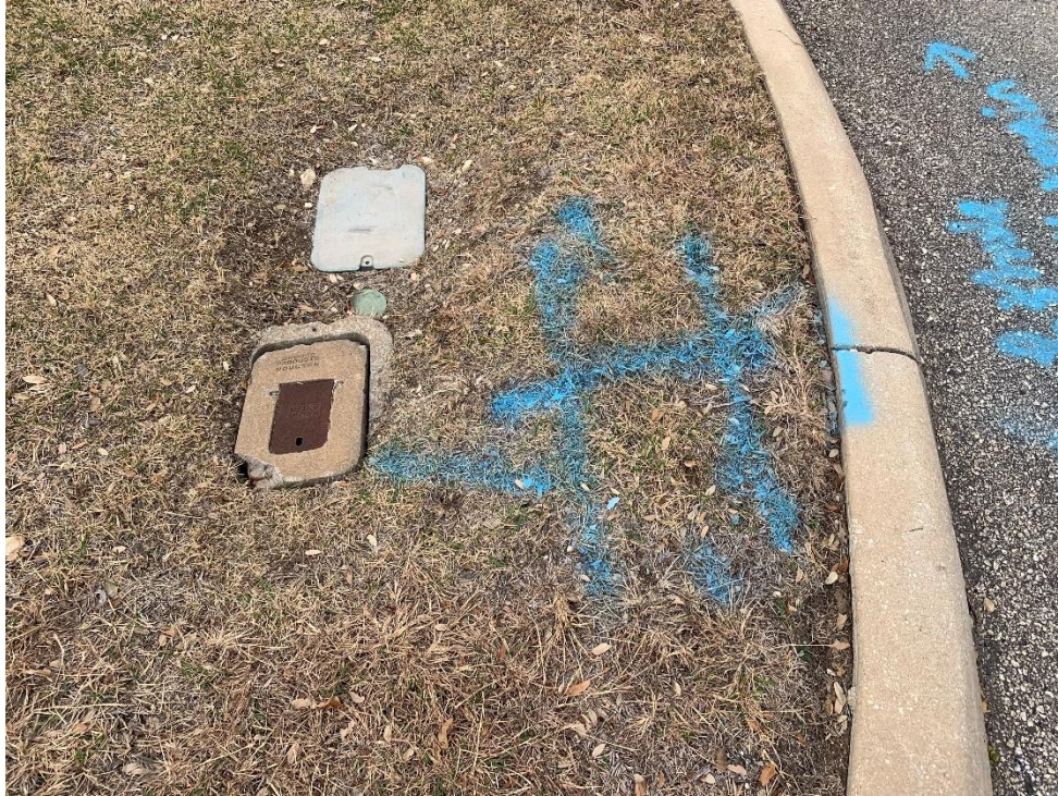
Photo #11: View of water meter box, suspected irrigation manways and marked utilities at the location of feature of feature S-7. Photo taken January 6, 2023.
