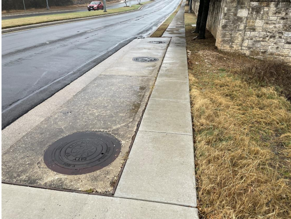
Photo #13: View of stormwater inlets at the location of feature of feature S-9. Photo taken January 28, 2023.
