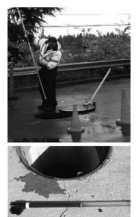
Inspection Utilizing Sediment Probe
