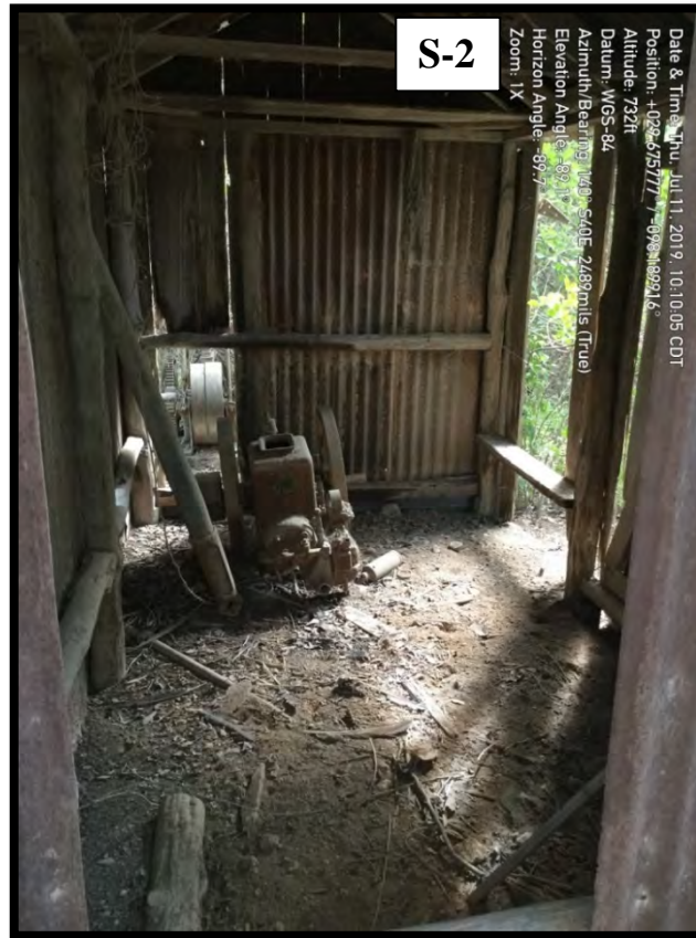
Motor in the pump house by feature S-2.
