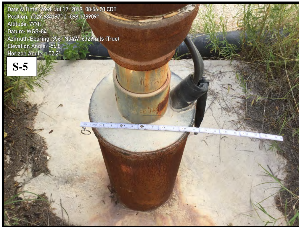
Concrete seal and surface slab on feature S-5.
