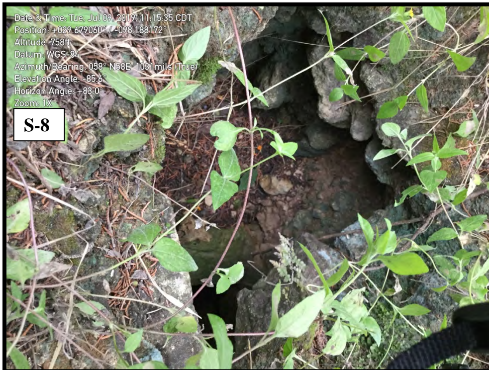
Large solution cavity in Zone S-8
