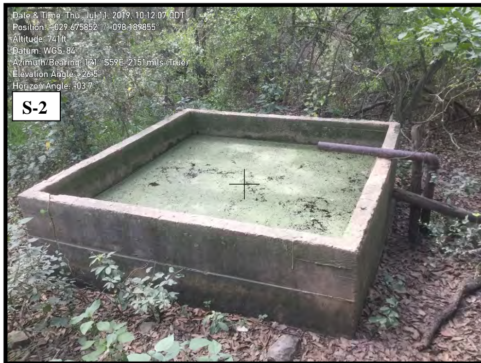
Water storage tank next to feature S-2.
