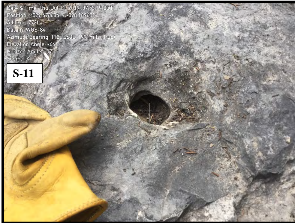
Feature S-11: Small Solution Cavity
