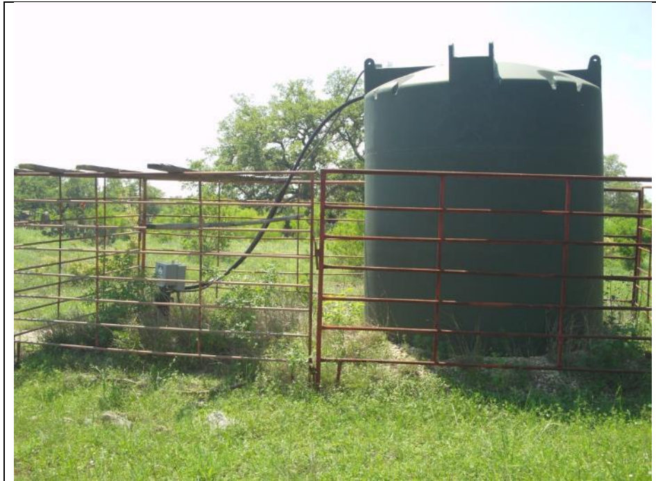
Photo 19: South Water Well (S-14-MB) - view to west
