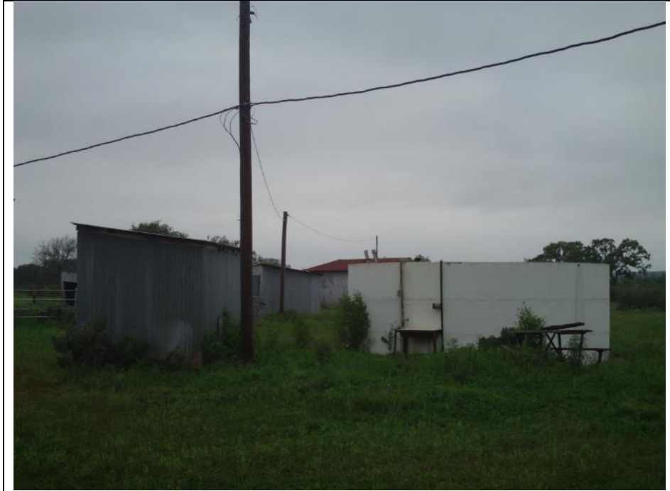
Photo 31: North Water Well (S-13-MB) shed and tank
