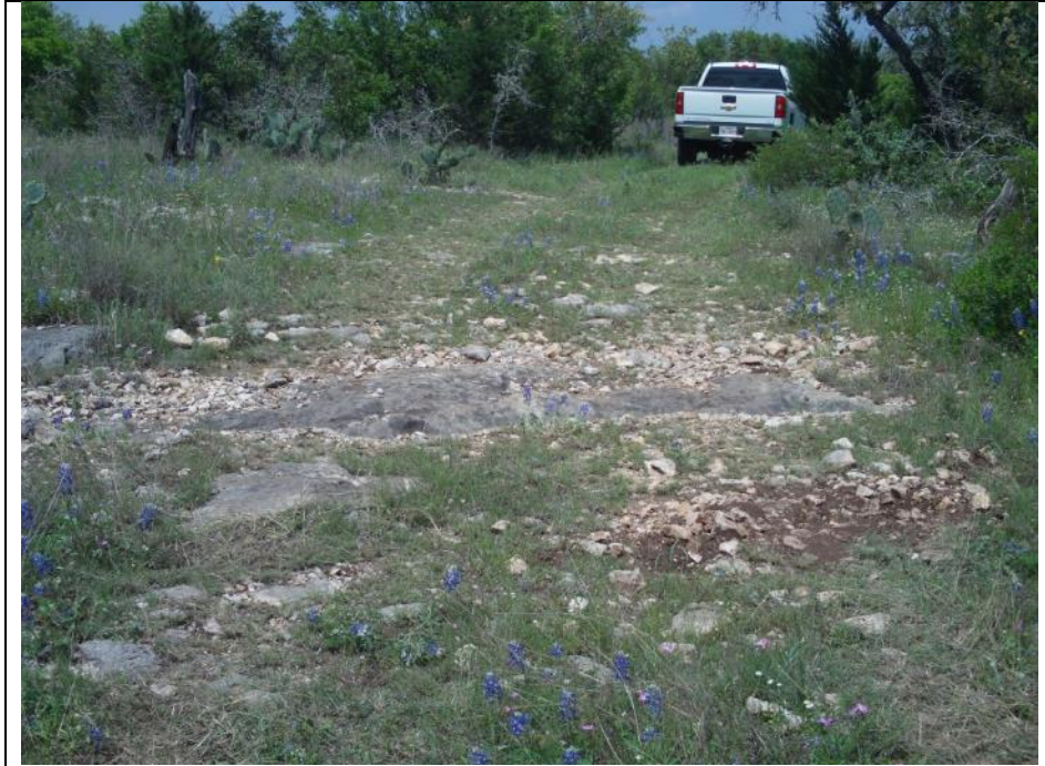
Photo 15: Limestone ledge indicates presence of fault trace (S-1-F) - view to northwest
