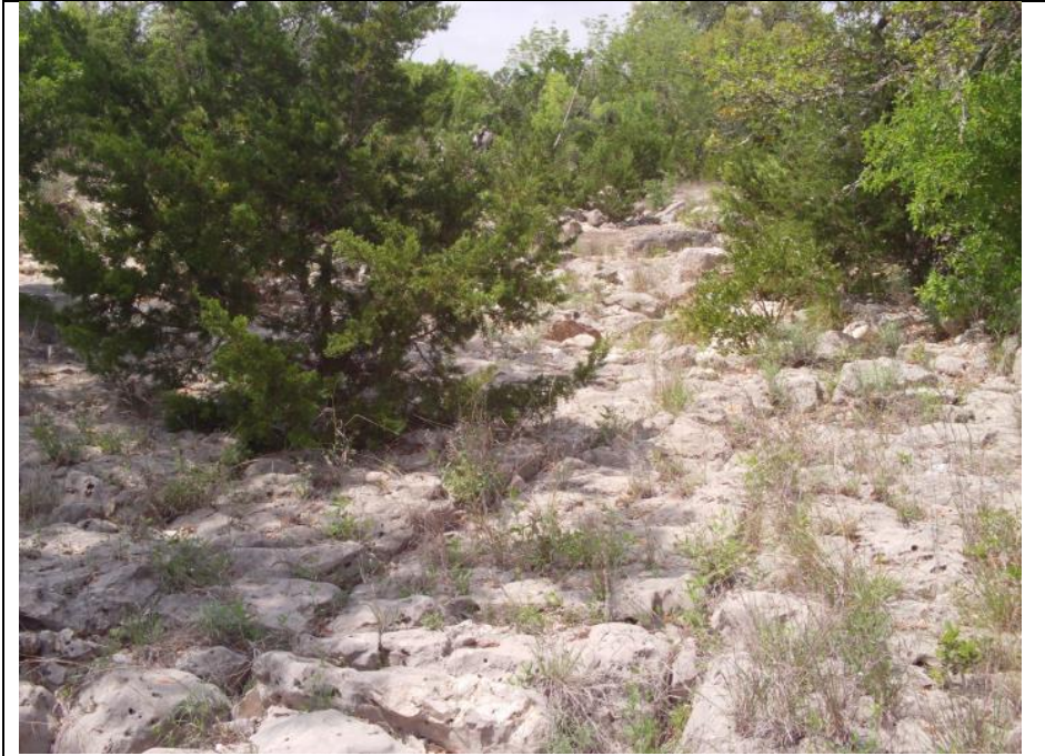
Photo 13: Gray fractured bedrock in tributary to Elm Creek – view to southeast (near of crossing of Fault Trace S-1-F and tributary to Elm Creek)
