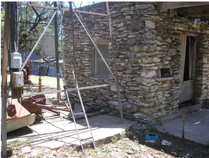
Photo #67 – View of the windmill associated with PRF #S-26 and an adjacent structure.
