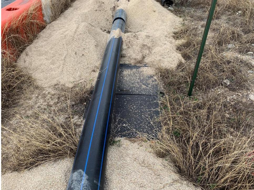
Photo #10: View of SAWS water line installation (feature S-10) and AT&T utility box (feature S-1).
