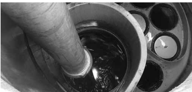
Vacuuming Sump Through MAW
